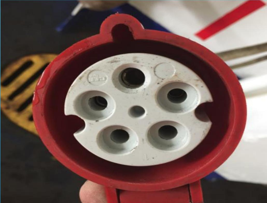
FOR ELECTRICAL SUPPLY 415V/50HZ/35A
